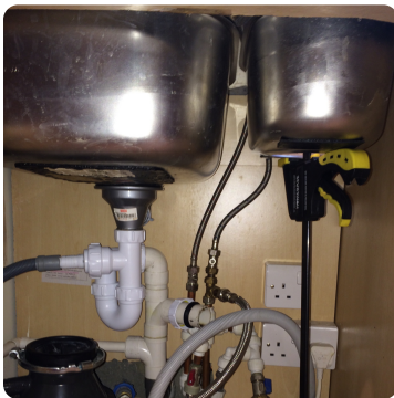
Caption Sink clamped in place
